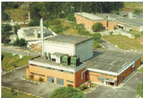
Figure 20. IPEN/MB-01 Reactor building
